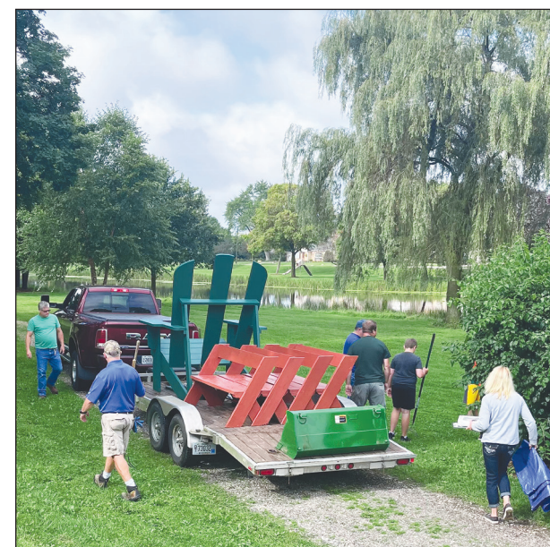
The large adirondack chair and benches built by Kewaskum Boy Scout Jake Gigstead are hauled into River Hill Park for installation.
