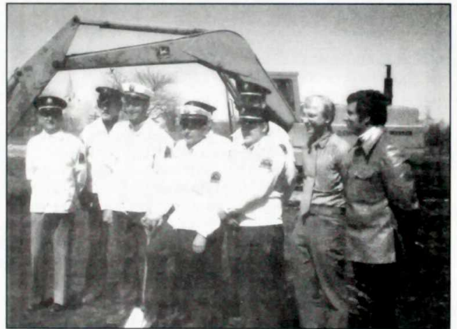
Grounding April 12, 1976 for the new station on Fond du Lac Avenue.
