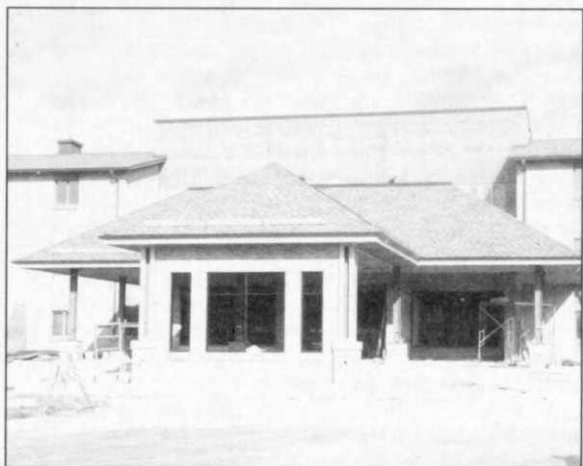
The new carport at the main entrance to Cedar Ridge is shaping up and should be ready for a November opening.
