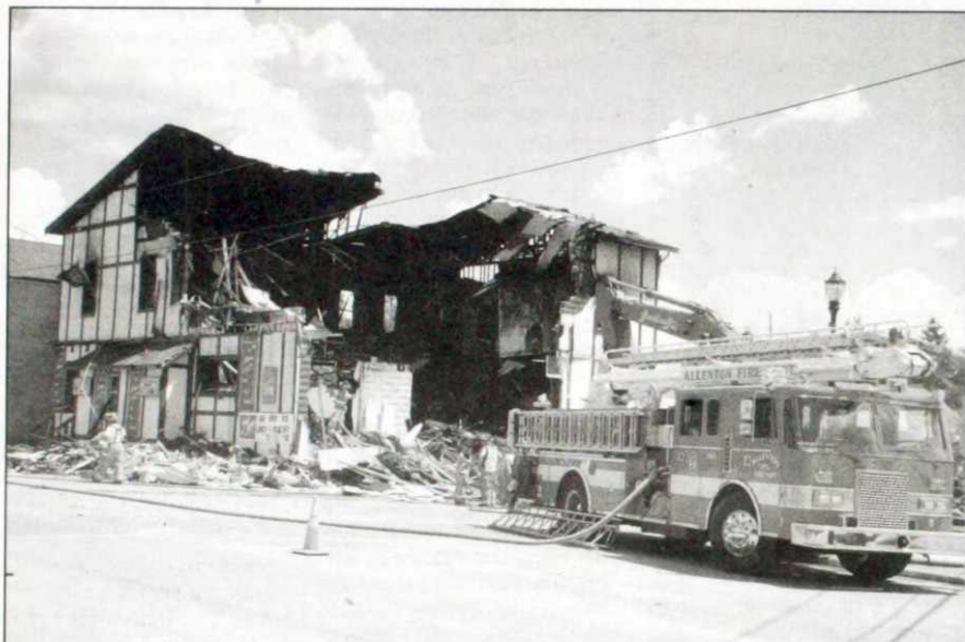
Allenton Firefighters among others remained on the scene of a disastrous fire that consumed The Allenton Inn on Highway 33 in the town of Addison.
