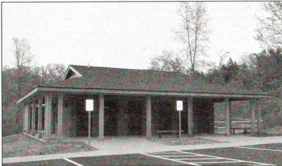
A view of the new shower/bathroom facility in the 300 section of Mauthe Lake Recreation Area.
