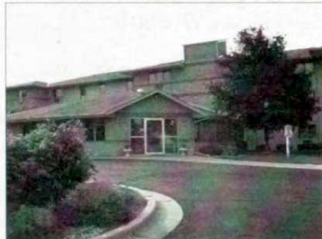
Maple Dale Manor of Kewaskum I Maple Dale Manor Apartments
