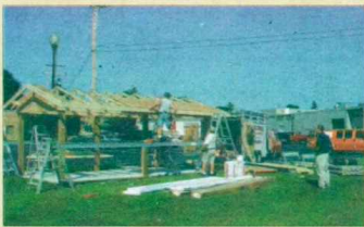
Construction in progress.
