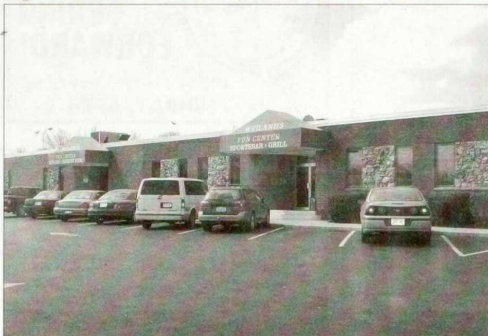
King Pin Lanes owner, Cary Serwe has joined a partnership that bought Weiland's Fun Center in West Bend. Serwe and Carter Smith will transform the bowling center into King Pin Bowl and Ale House. Renovations are expected to start in May.
