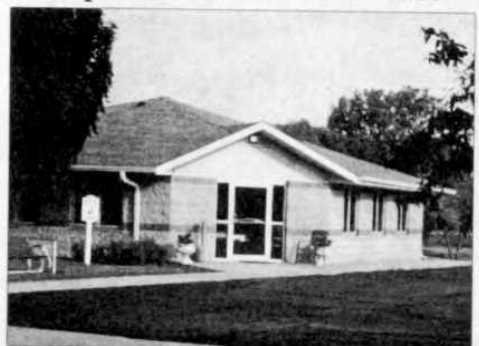
Maple Dale Manor of Kewaskum II 14-Unit CBRF
