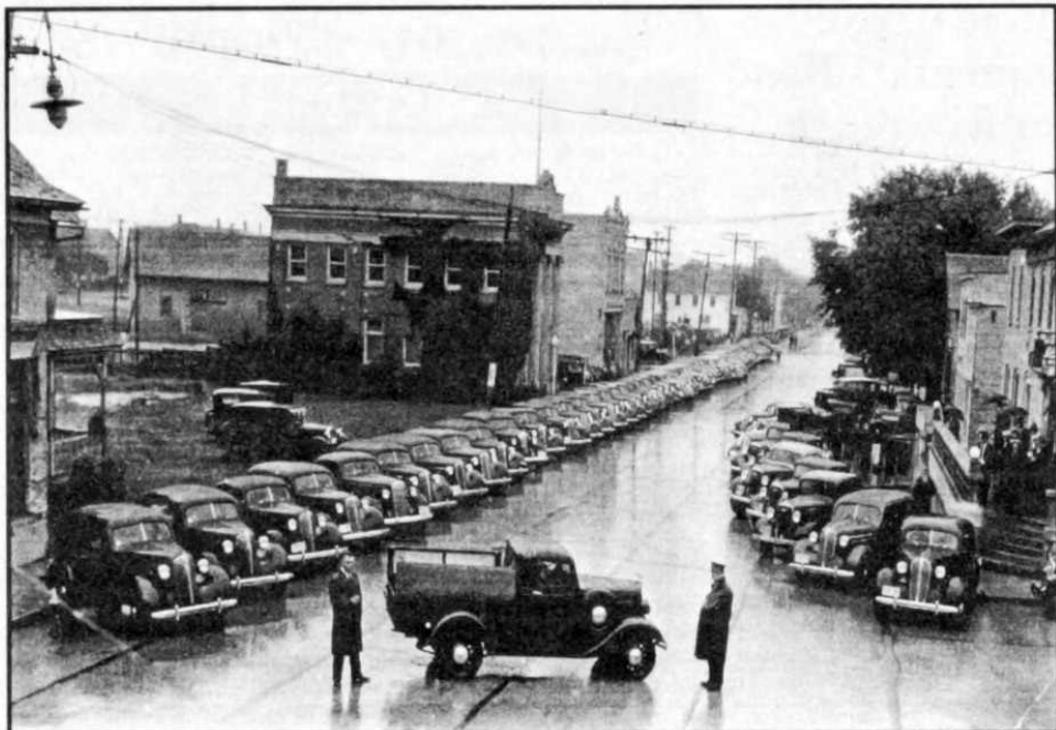
One hundred-six Chevys from the Kilian Honeck Chevy dealership lined both sides of Main Street in Kewaskum in 1936 according to information recorded on the back of the above photo. The buildings shown in the picture include a partial view of The Republican House, on the right, which now houses Woody's Steakhouse, and the Corner Drug Store on the left, which is now occupied by the Coffee Corner. In the center of the photo, left side of the street is the Bank of Kewaskum and the H.J. Lay Lumber Company which were both razed many years ago.
