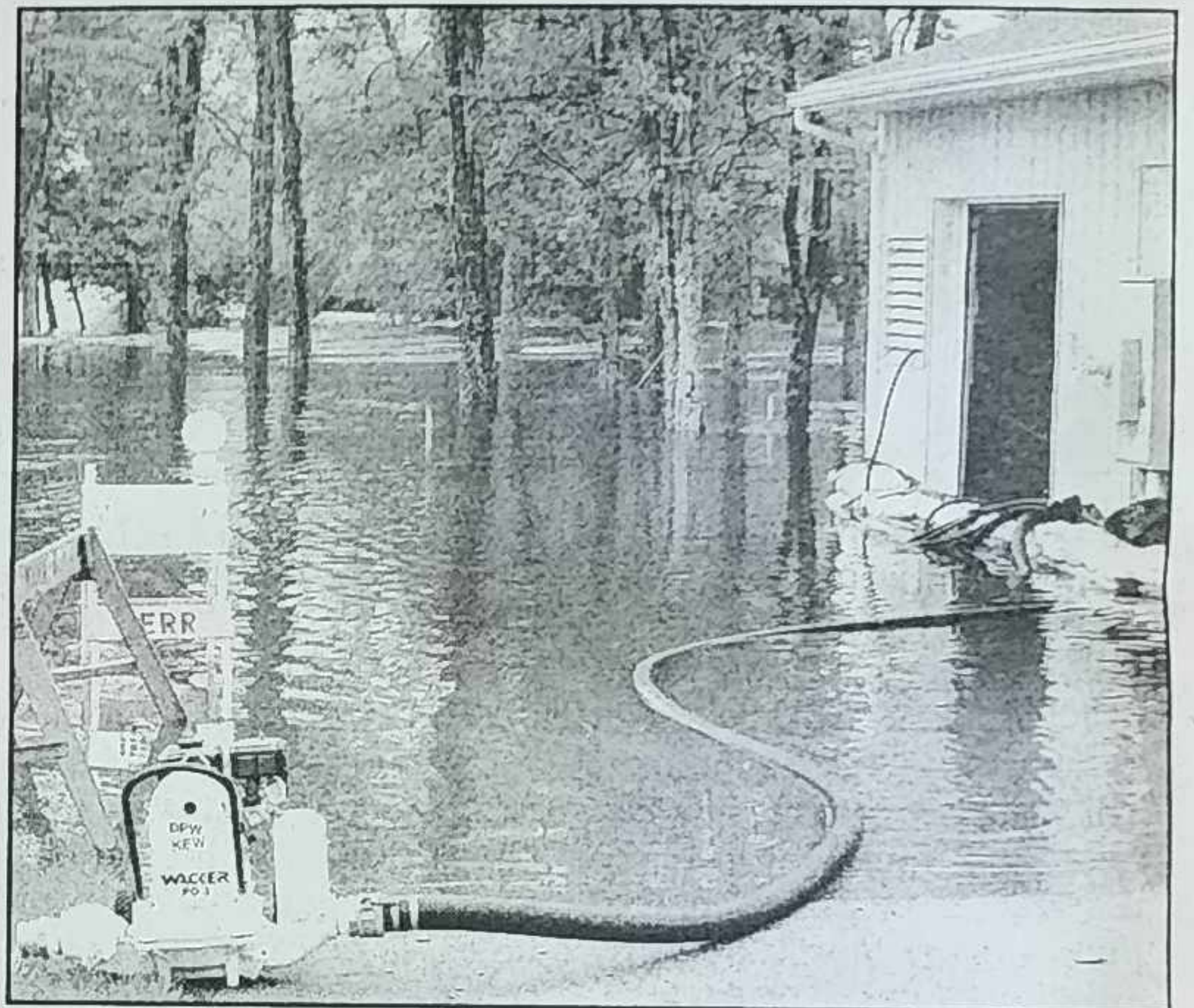
Kewaskum Wastewater Management crews were forced to sandbag and pump water out of the pump-house located in River Hill Park. Former DPW director Augie Bilgo stated Saturday morning the last time flooding of this magnitude occurred was in the spring of 1989 when the ice melted. It is unknown the last time River Hill Park flooded due to extreme rainfall. Bilgo shared a collection of photos from that time period with this newspaper. Due to space constraints they could not be published this week but we hope to bring them to you in the next edition. Anyone with older flood pictures or memories are asked to contact Andrew at 262-626-3312.
