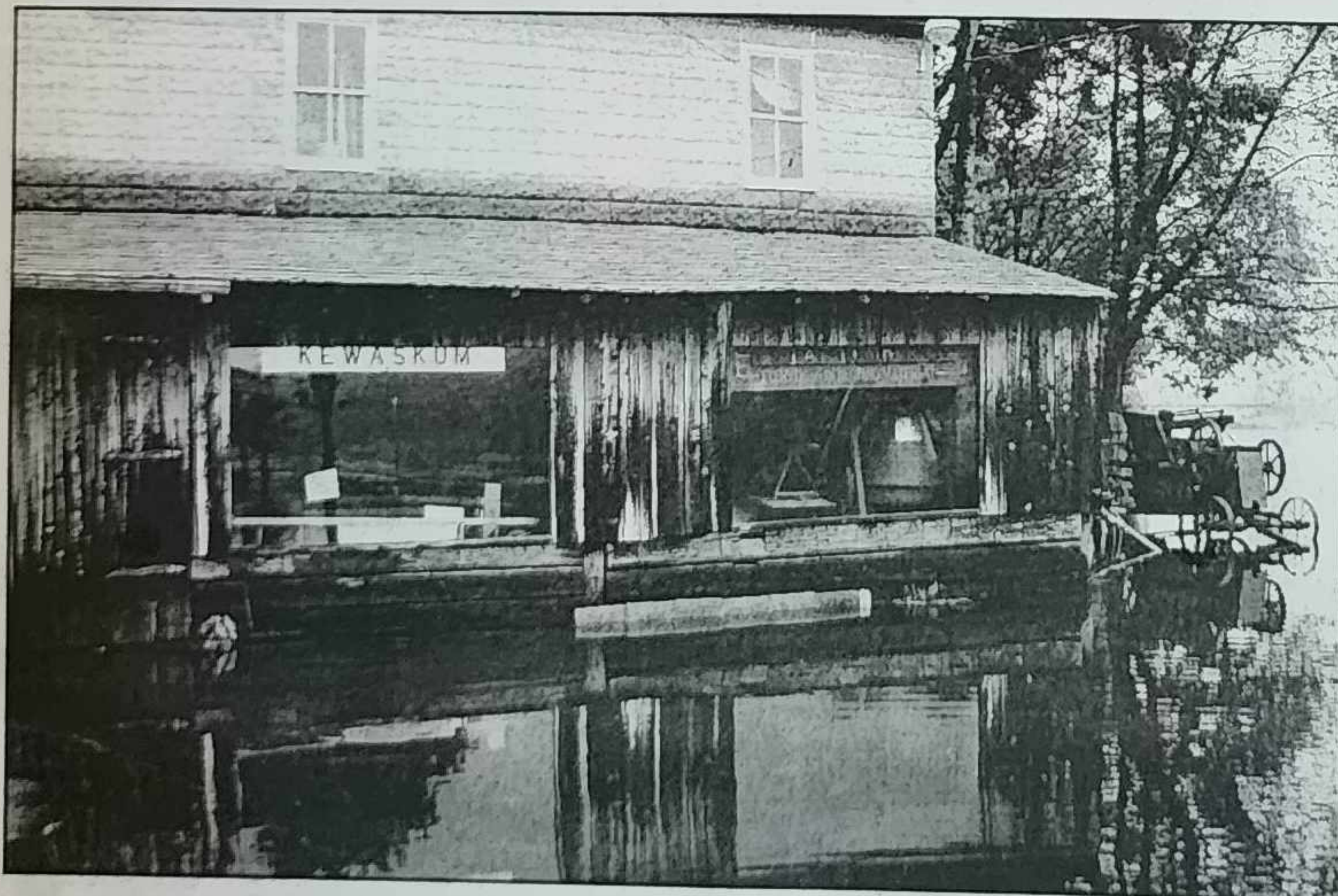
The Kewaskum Museum also sustained flood damage but according to Village Administrator Dan Schmidt nothing was destroyed. Schmidt indicated that about 8-10" of water flooded the basement of the log house and museum. The DPW piled sandbags in the interiors to stop further flooding.
