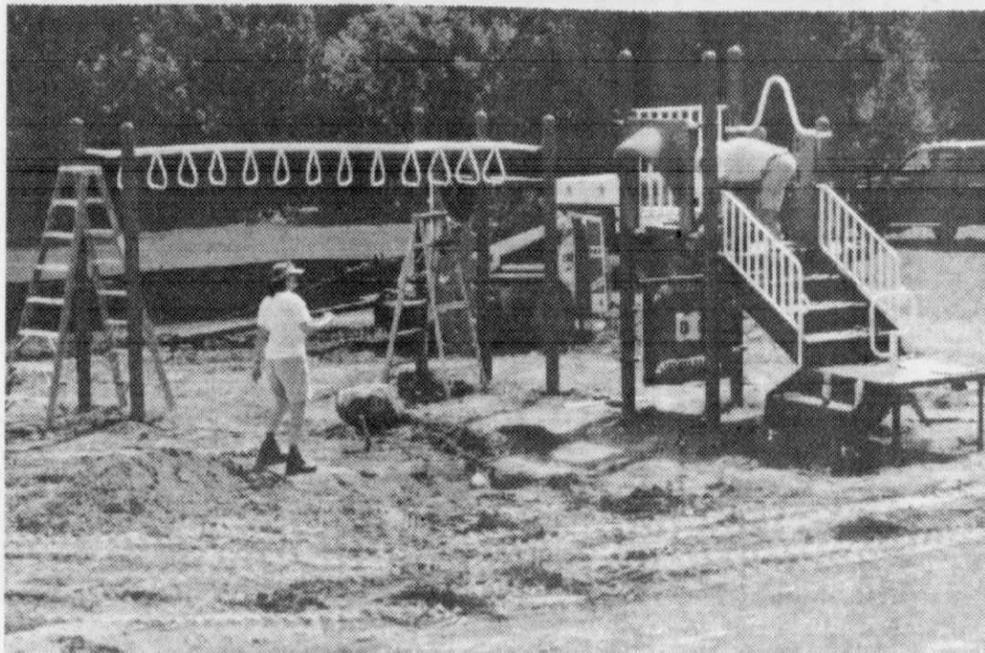
The new playground equipment being installed at St. Lucas.
