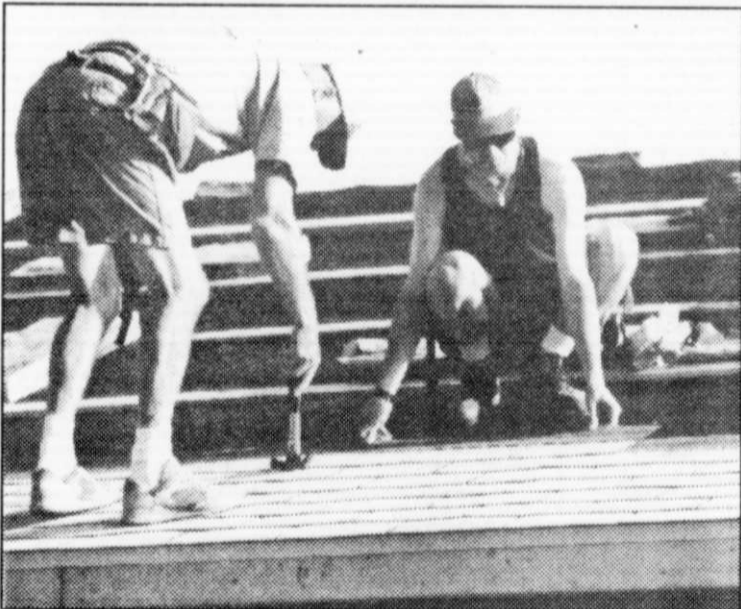
Mark Steinhardt (left) and Pastor Eric Kirkegaard working on the roof.
