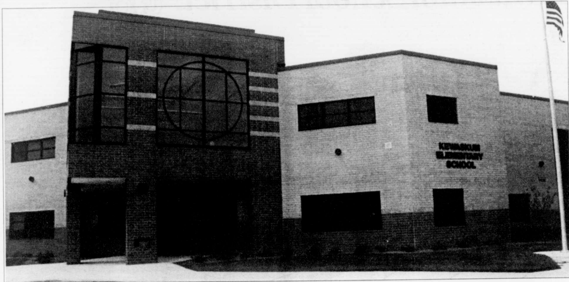
A front view of the newly constructed Kewaskum Elementary School
