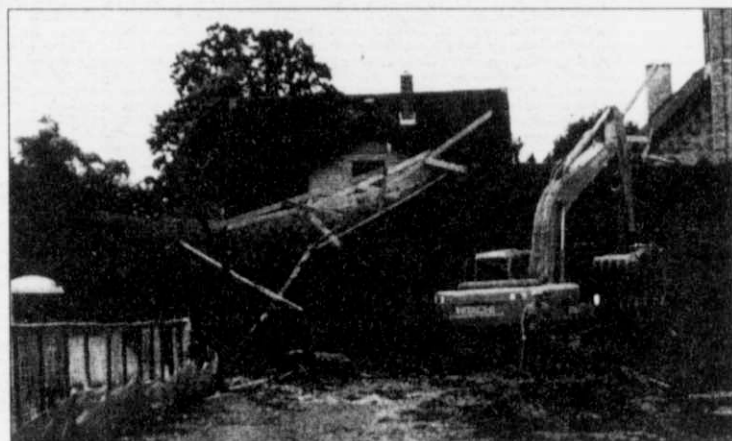
A view of the grandstand at the former baseball field being demolished.
