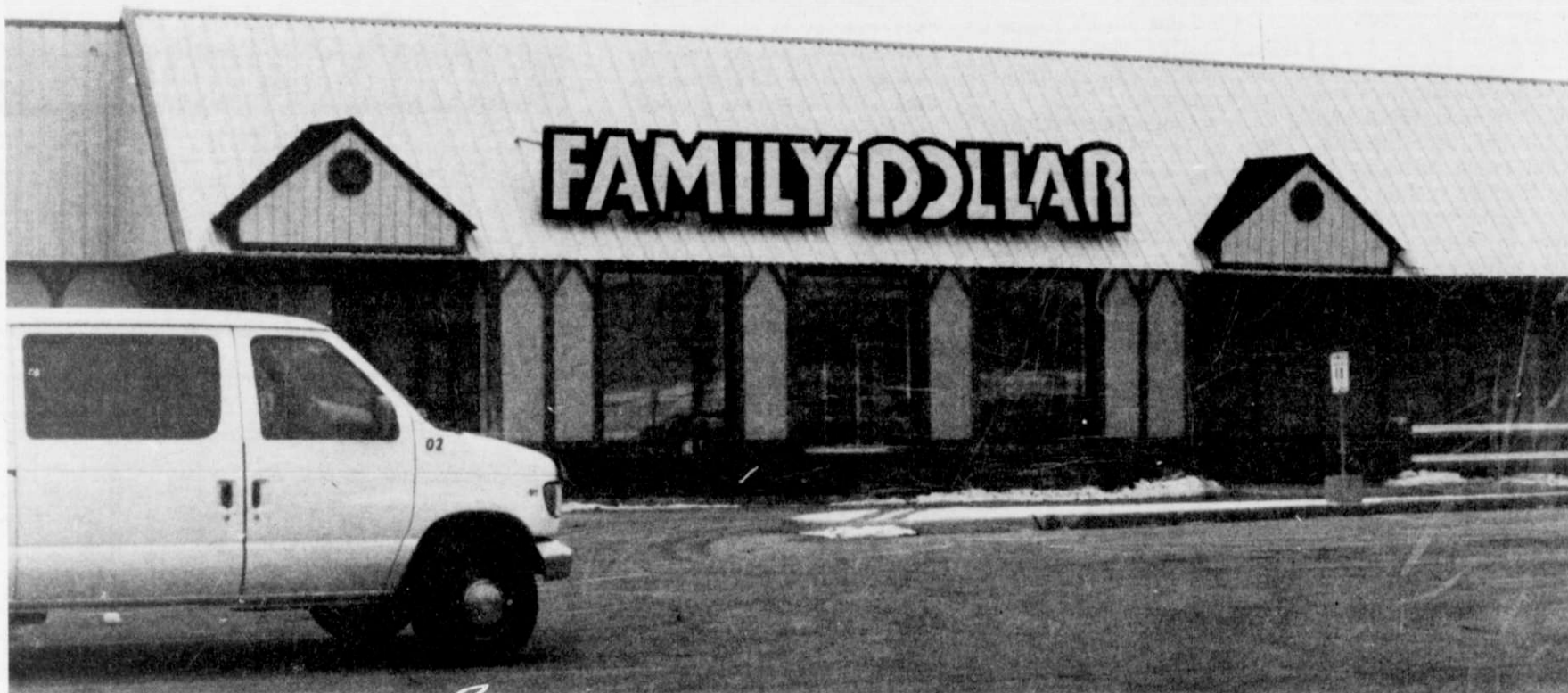
The new signage for the Family Dollar Store was installed this past week. The store is scheduled to open in the Kewaskum Mall on March 1. Crews have been kept busy getting ready for the arrival of shelving and merchandise.
