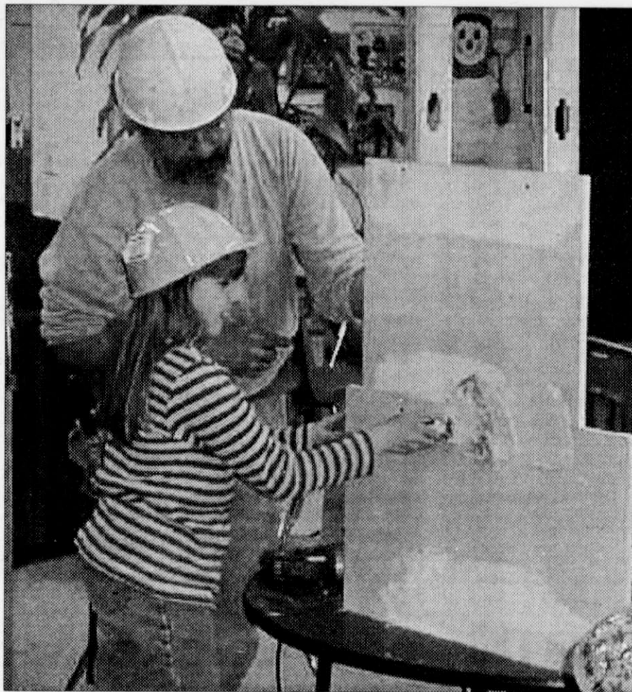
Katie Peters, a fifth grader at KES learns first hand how to apply drywall mud from "Carpenter Bob" a C.D. Smith construction worker. Students from KES have been touring the school and learning how their school is being built.
