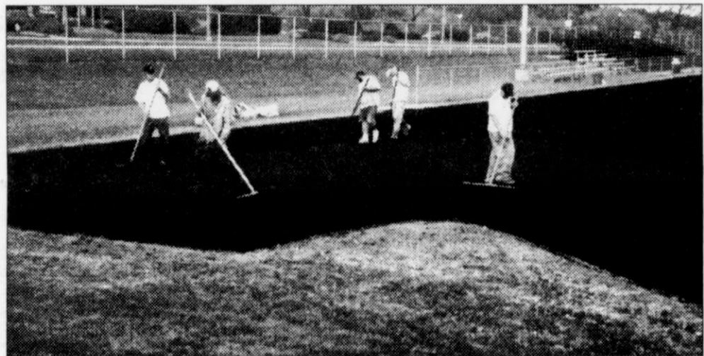
Workers from Athletic Field Services of Genesee Depot, Wisconsin, spread the fourth layer of rubber particles on the Kewaskum High School track prior to the spraying of liquid latex binder and sealer later in the day. A total of six layers of rubber particles and liquid latex coats were applied to the track.
