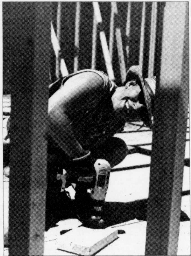
BE CAREFUL MARY!! Mary Schoofs shown installing floor boards.
