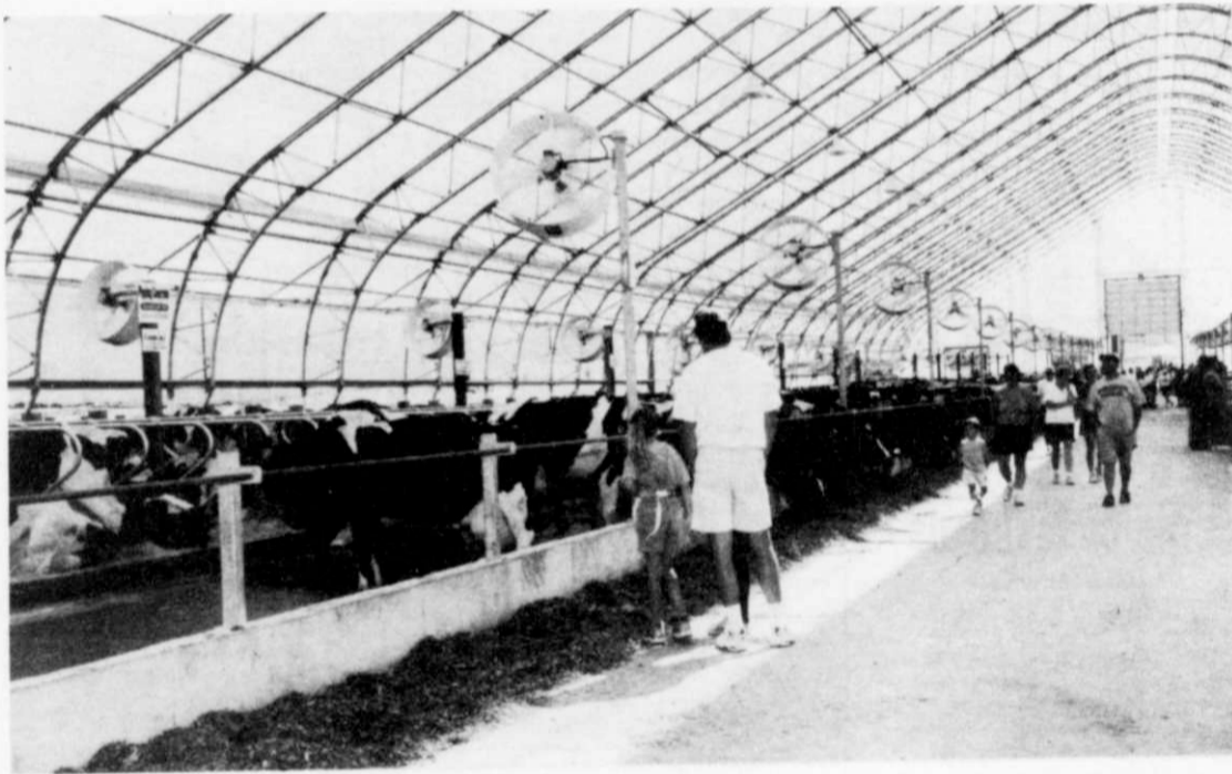
Visitors to Farm Progress Days had the opportunity to walk through one of the new canvas-covered barns on the Allen and Carol Abel farm. The family has undergone a major expansion to improve their operation and be able to accommodate the large herd of 1200 cows.
