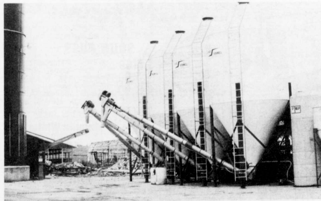
Among the many improvements made on the Abel farm are these bottom-augured feed tanks used to store feed for the huge dairy herd and replacement animals
