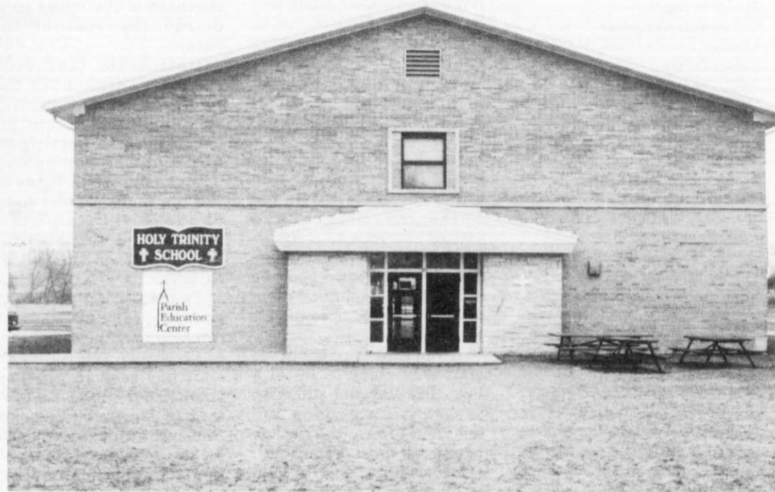
The Holy Trinity School expansion project, tentatively scheduled to begin in March, 2000, will be erected onto the front (north) of the building on the grassy area that is pictured above.
