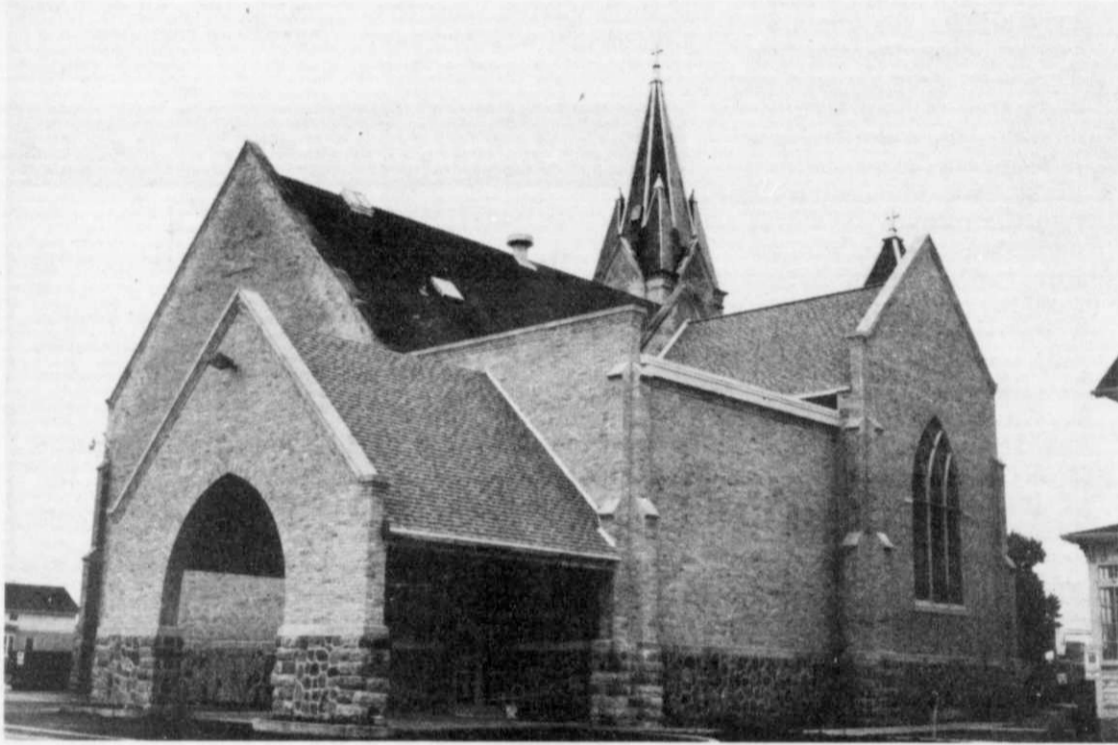
Shown above is a rear view of the renovations made to Holy Trinity church. The new, attractive carport provides a handy dropoff point to parishioners during inclement weather.
