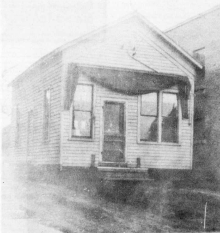
This was the temporary location of the Yoost Butcher Shop while the new building was being erected.
