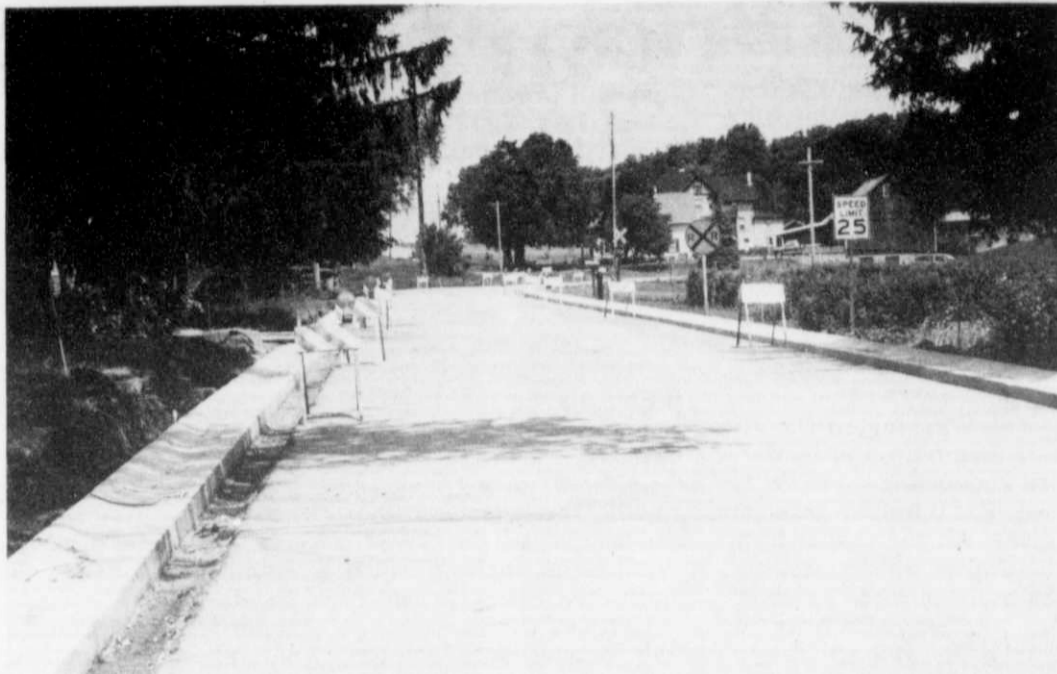
Summer road work has begun in Kewaskum. Curb and gutter and sidewalk were added to Old Fond du Lac Rd this past week, also getting a facelift was the access road off STH 45 north of the village. The project cost taxpayers $80,000. T.P. Concrete of Fredonia sees the project being finished by August. Statesman Photo: Andrew Kuehl
