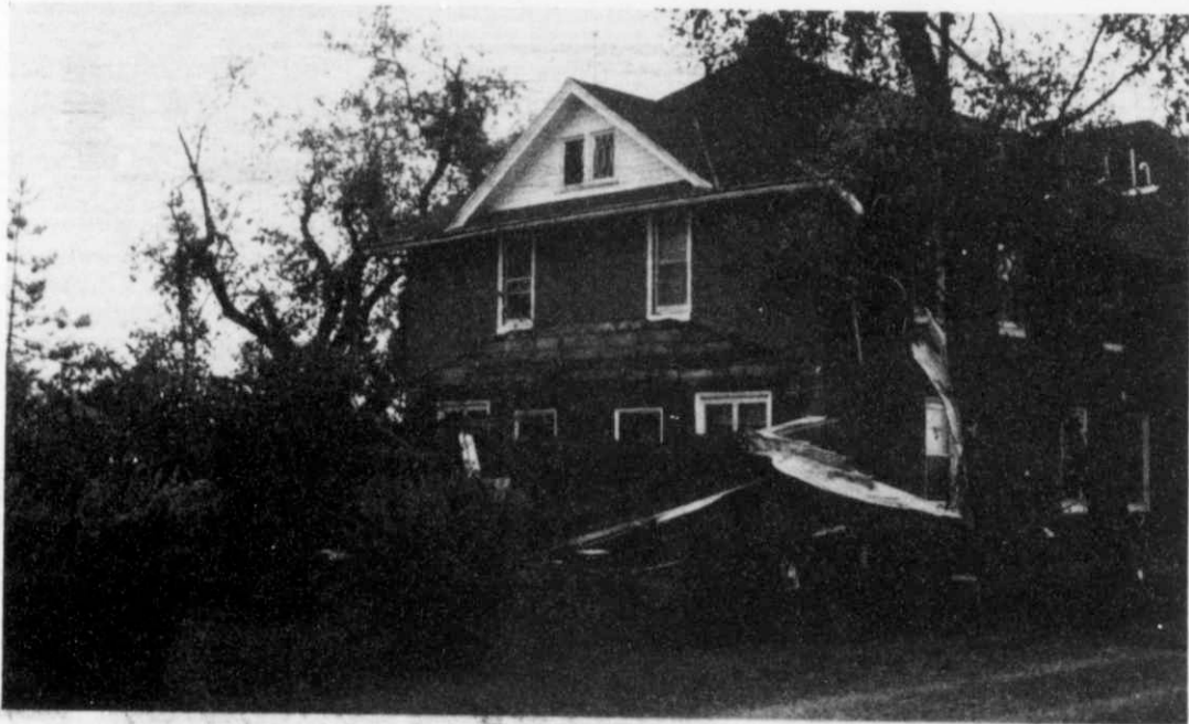
A bevy of branches and limbs destroyed the porch of this Town of Auburn home. Rubble from a neighbor's barn can be seen in the background.
