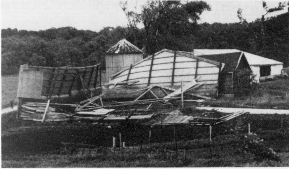
A destroyed pole building on Mill Road in New Fane.
