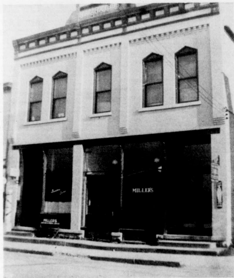
The building where Tan-Talizer Tanning Salon is now located is the next stop on our "Stroll Down Main Street," traveling east on the south side of the street. Our sources tell us that at one time it was the Clem Reinders Furniture Store and later the Miller's Furniture Store (as shown in the photo nearly 50 years ago.) The building was also "home" to the Frank Felix Radio Repair Shop in the rear and the Hubert Wittman Barber Shop.
