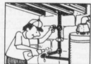
If you suspect you have a gas leak, do not light a match to try to spot it. Instead, lather the suspected area with soapy water so that the escaping gas will cause bubbles and pinpoint the danger area.
