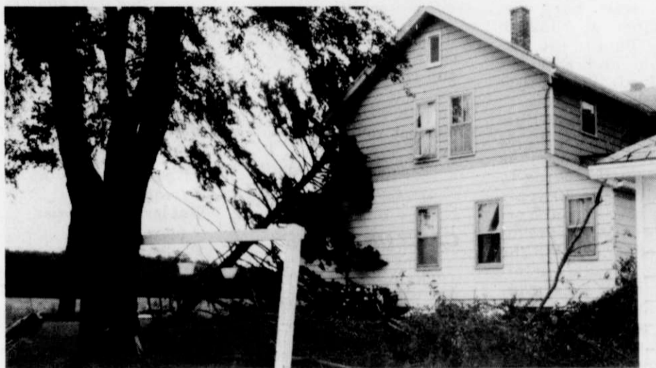
It is obvious by the above photos taken of the front and rear of the homestead on the Floyd Klug farm located about eight miles northeast of Kewaskum, that a tornado either touched down or was very, very close. The large tree in the front yard was literally torn from its trunk and laid up against the roof and side of the house. Large limbs were also strewn up against the house in the rear. Another huge tree in front of the Irvin Lepp farm in the same area was snapped off and had to be cleared off the road. The storm's fury was also witnessed in the cornfields in the area that were flattened.
