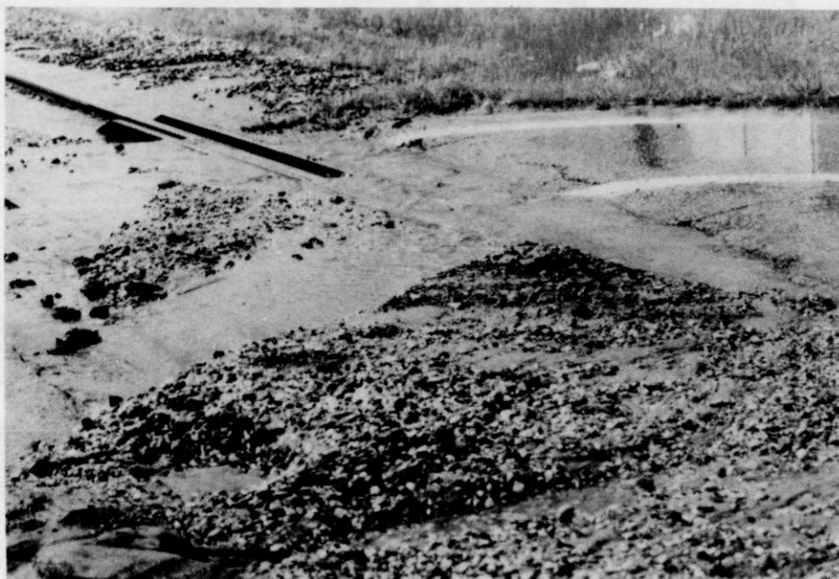
Shown above is the water, gravel and sand that washed over the railroad tracks shortly after the main line break was discovered on July 4th.
