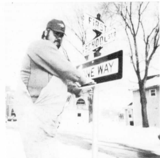
One Way signs for School Street were installed Tuesday afternoon by village crew Lead Operator Alan Kuehl.
