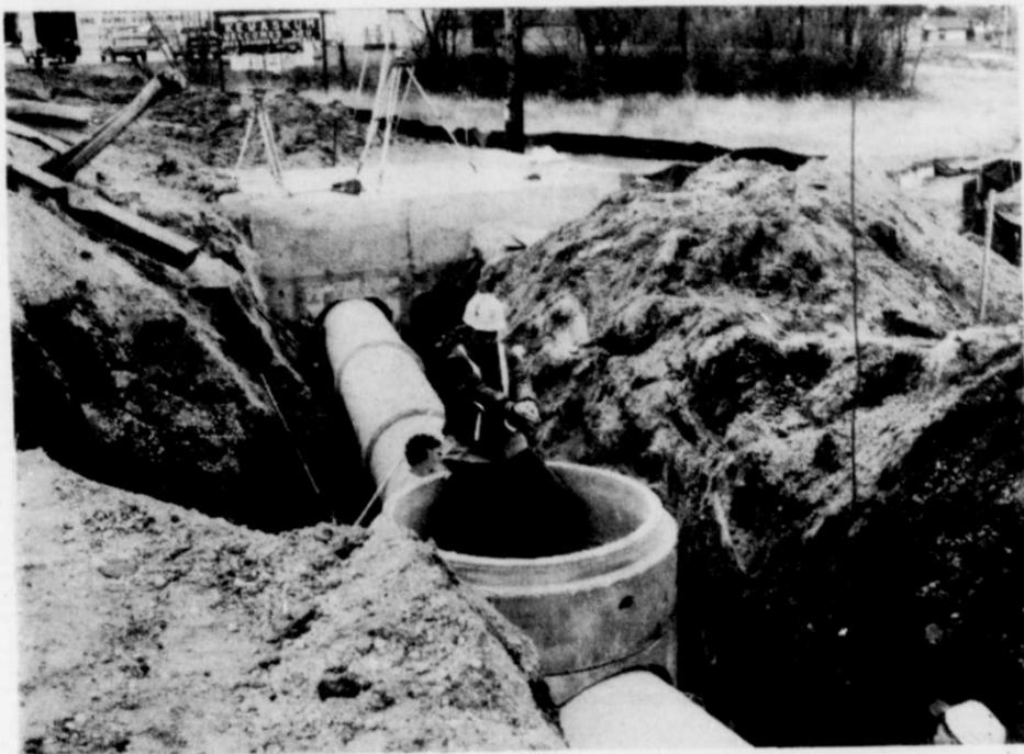
Work is progressing rapidly on the Wisconsin Department of Transportation Highway 45 project running through central Kewaskum. The storm sewer installation on the north end of Kewaskum is shown above as the pipes are being placed into the manhole. Masson Brothers, Inc. of Rhinelander are the contractors. The west half on the north side of the curb and gutter and asphalt paving is expected to be finished within approximately two weeks which should open the west half of the road to traffic.
