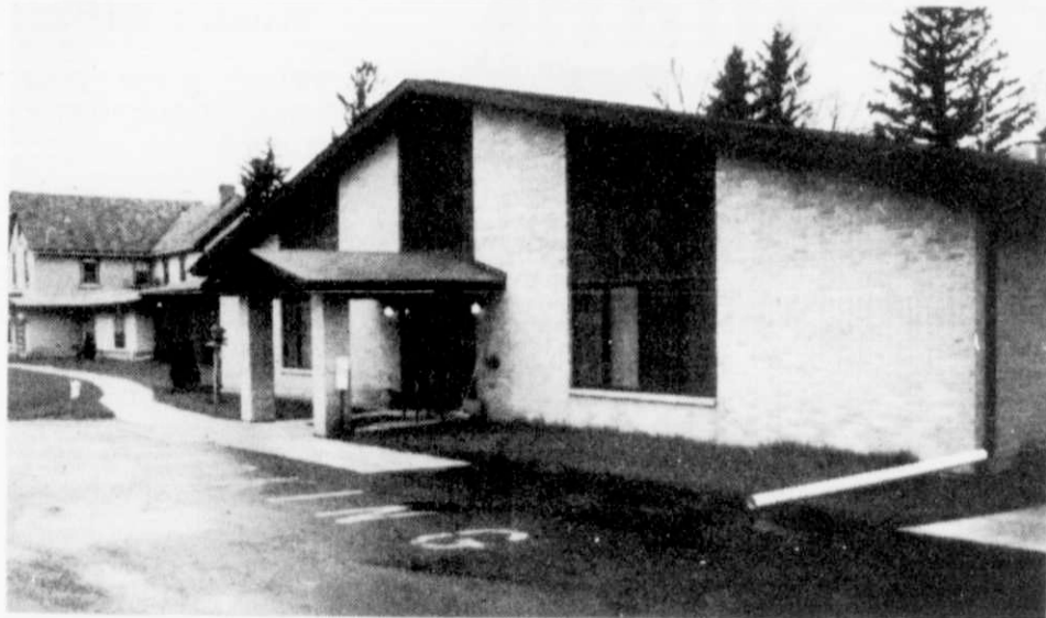
The Beechwood Rest Home facilities.
