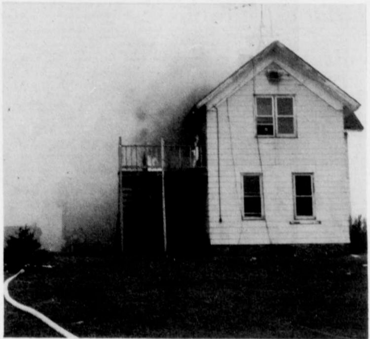
Shown above is another view of the duplex in rural Boltonville that was gutted by flames on Monday morning, after the flames had quickly spread to the upper level.
