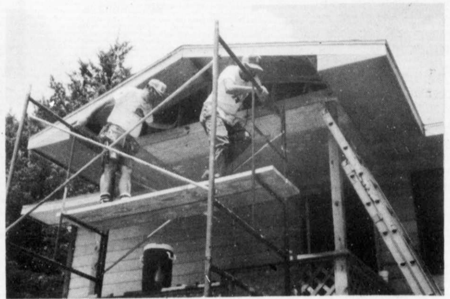
Steve Van Ess and Clark Pearson on the scaffolding.
