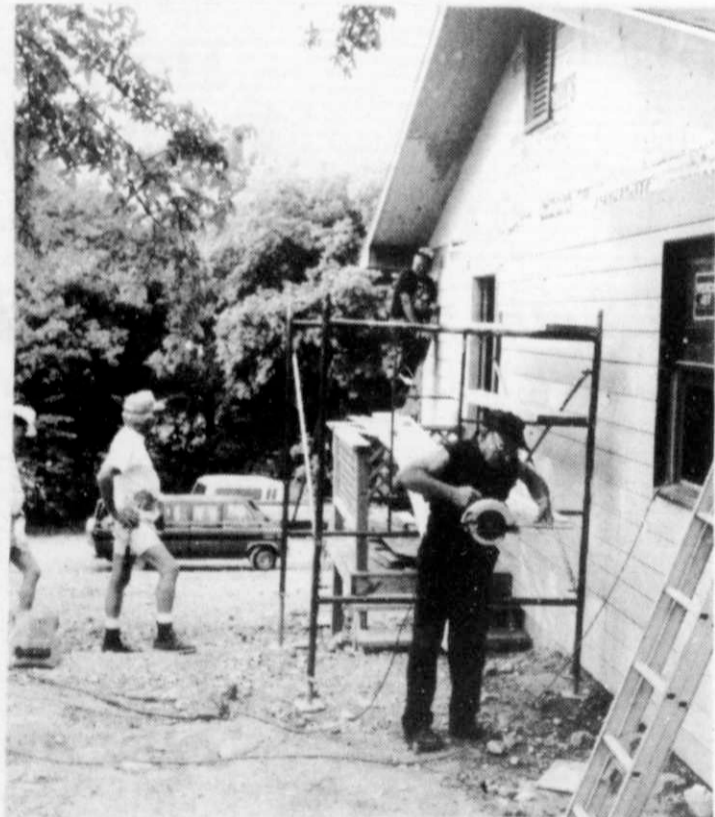
Richard Zarling, Willard Gruhle and Clayton Stautz working on the exterior.
