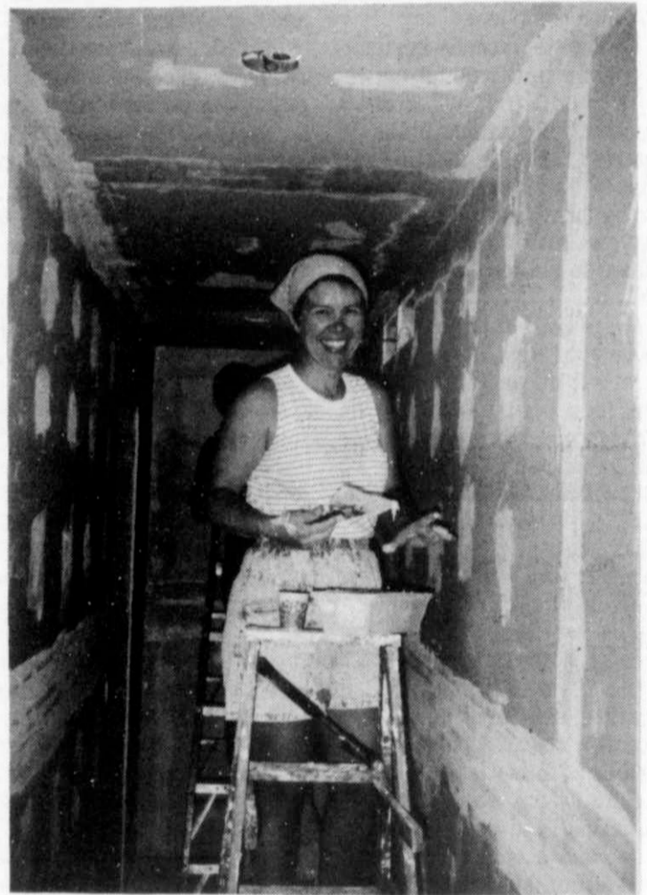
Gayle Van Ess dry-walling inside the house.
