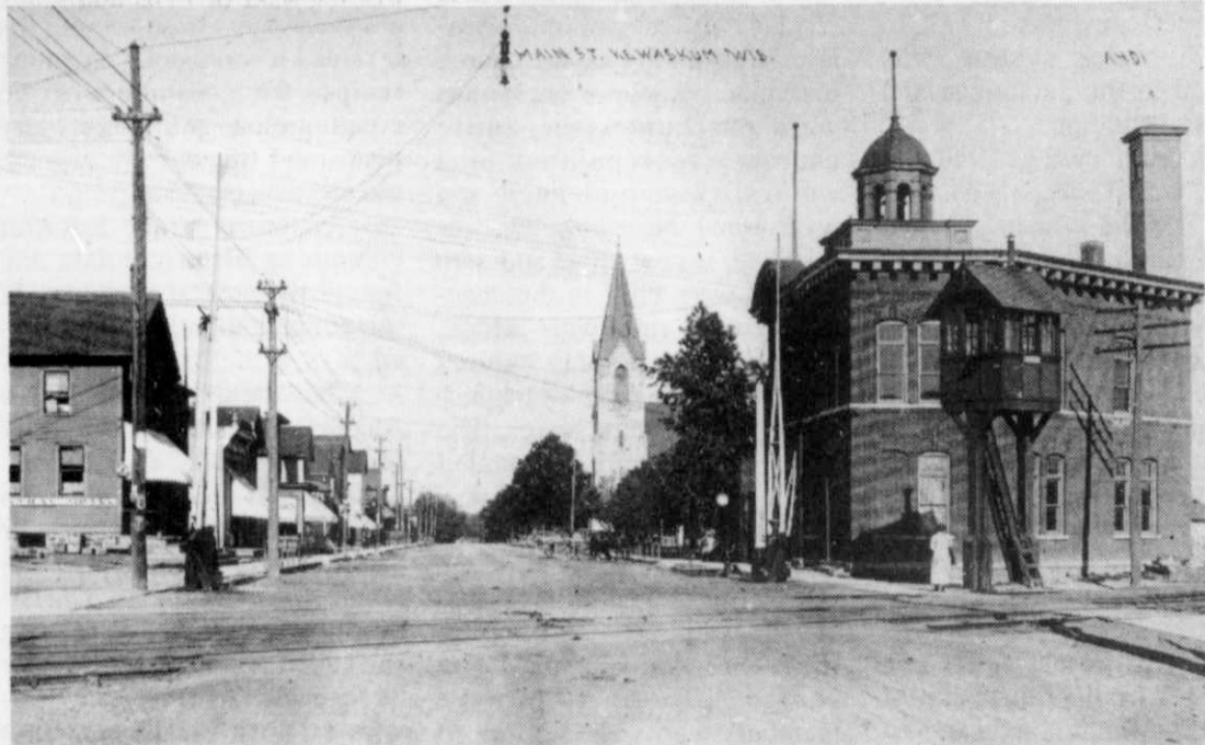
The above early 1900's postcard of Kewaskum shows the gate tower which manually controlled the gates as trains approached or left Kewaskum's depot.
