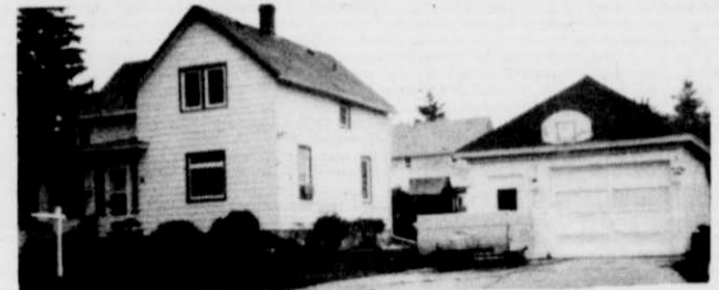
136 Elm St. East of Hwy. 45 - South end of Kewaskum 3 bedroom, 2 bath, 70's
