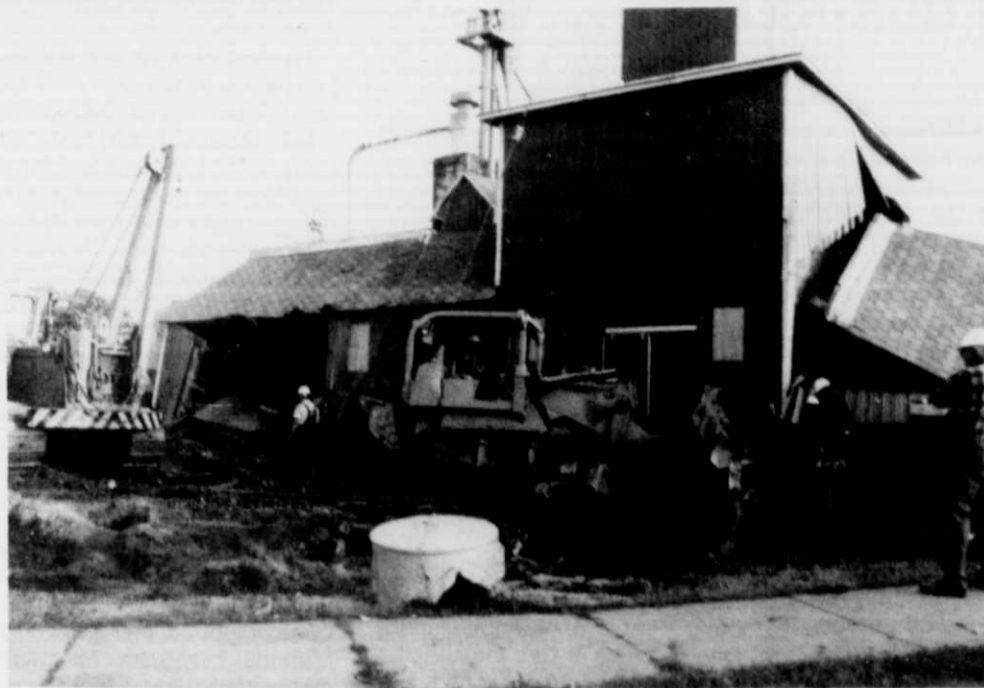
Crews worked to remove some of the derailed cars along side the damaged Eden Farm Supply feed mill.
