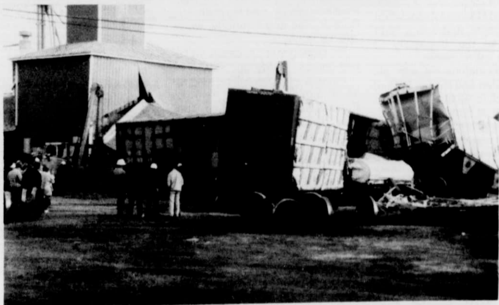
FRVR workers and spectators surveyed the damage. The car to left tore off the front of the mill. The cars to the center and right were just part of the sixteen car derailment.
