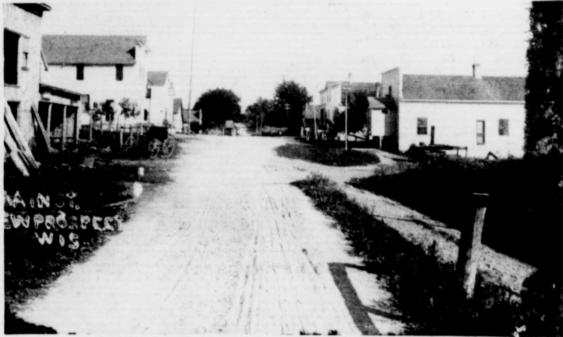
This memories picture of New Prospect was taken in the early 1900s. Its original name was Jersey. The first building on the left was built for a shelter for the horses when people came to town. The next building was Jack Welch's Tavern; today known as the Everglades. The next building was John Tonn's Tavern; today it's the Fin and Feather. Next building was Joe Uelmen's blacksmith shop. On the right was a cheese factory which burned down in the mid-twenties. It stood where the Black Angus stands today. The next building was a grocery store which was also destroyed by fire. The grocery store of today you can see in the distance.
