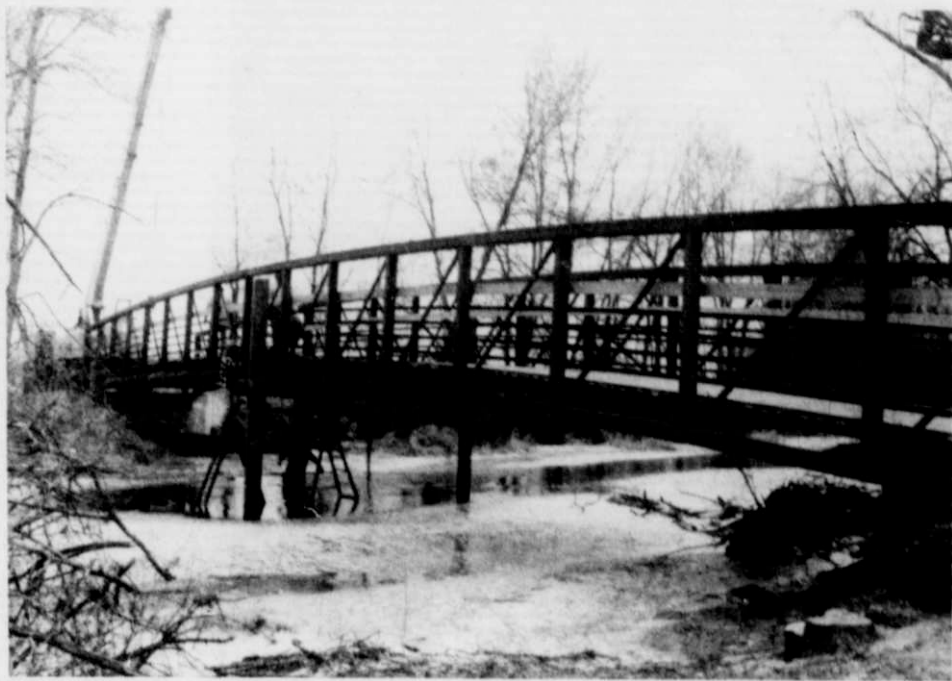
Runge Employees bolted the two sections of the 12 x 100-foot bridge together. The new bridge now connects the north and south sides of Columbus Park, providing not only a snowmobile trail link but year-round access of the entire park for other recreation enthusiasts.
