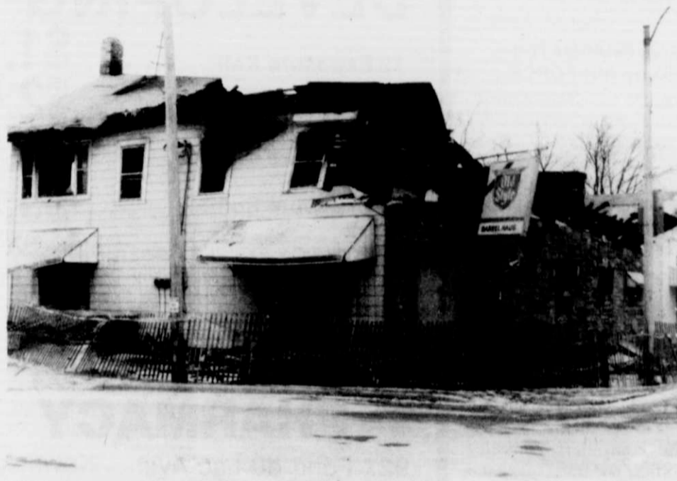
The landmark Barrel Haus building, like other century-old Kewaskum structures, will soon be a part of the past when wrecking crews move in to clear away the remnants of the January 14 fire.
