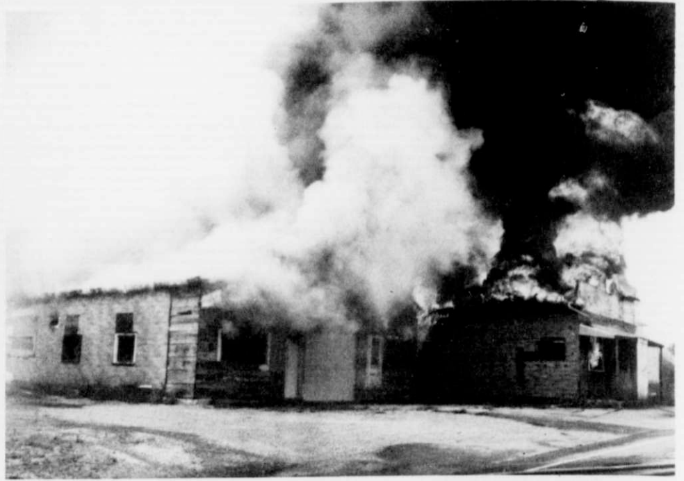
Smoke and flames billowed from the buildings.
