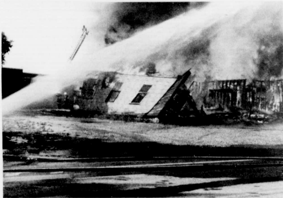
The walls of the garage collapsed in flames as Kewaskum's Tele-squirt (background) hosed down the St. Michaels School building at the rear.
