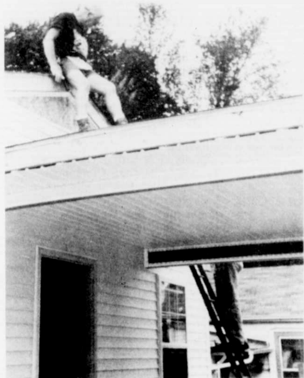
Richard Zarling completing siding on Habitat House in Lexington.
