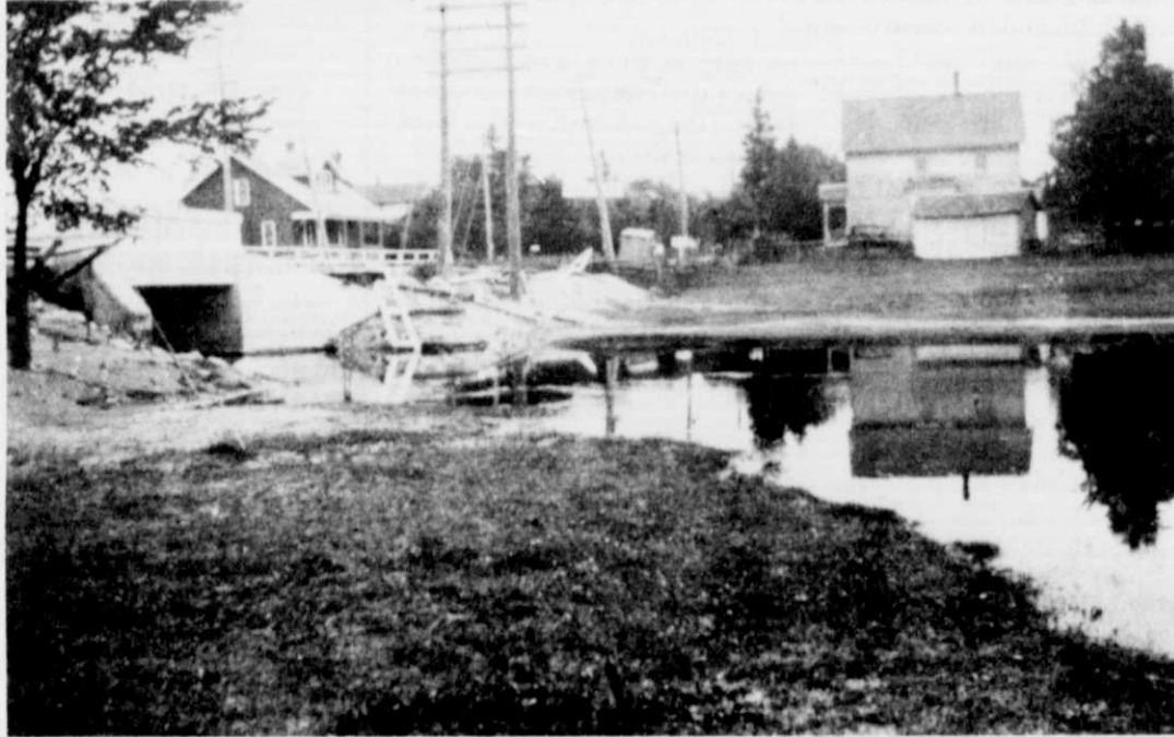
The Kewaskum bridge on South Fond du Lac Avenue, after the flood of August 3rd and 4th, 1924, 67 years ago. The picture was taken facing north, a week later after the flood waters had receded.
