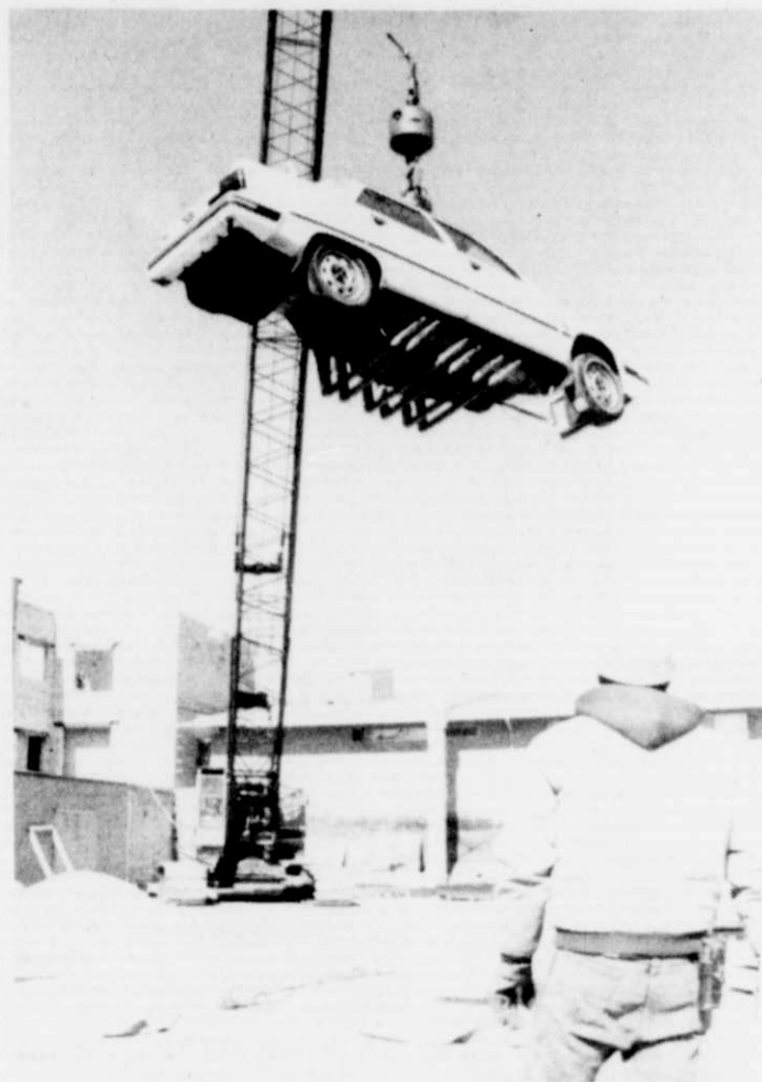
A crane lifted the car to its new home in the Cedar Haven Rehabilitation Agency Clinic in Fellowship House on the Cedar Lake Home Campus.
