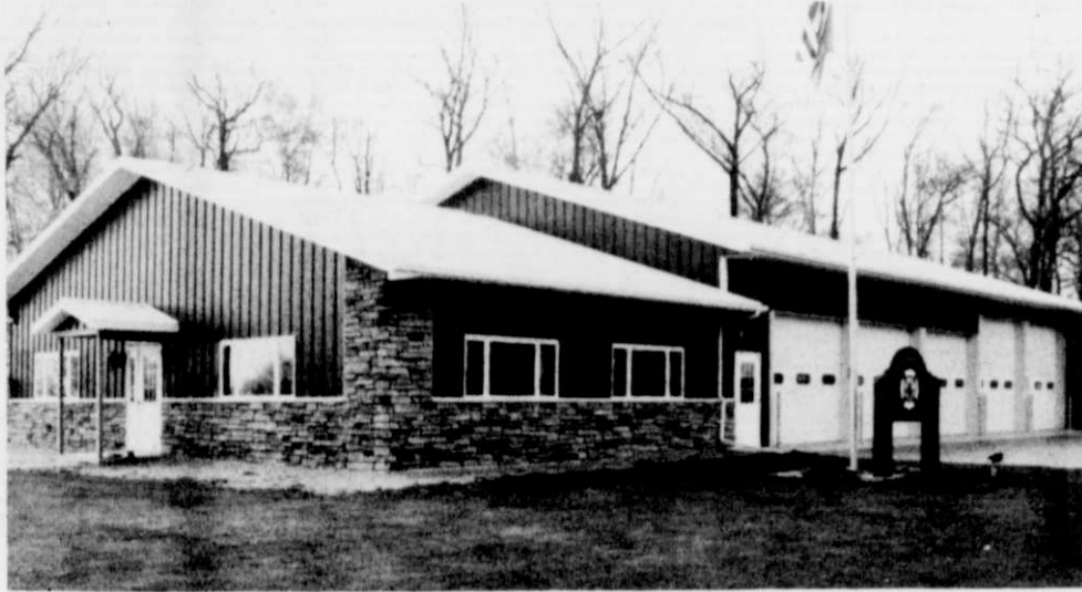
The recently completed Beechwood Fire Department meeting room, left, will be dedicated during the open house Sunday afternoon.
