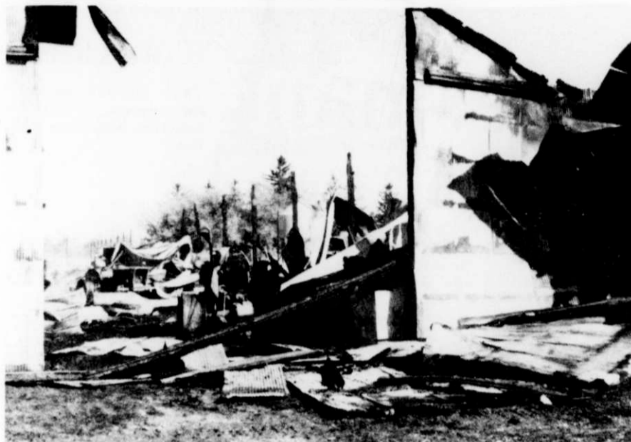
More than four hours later the last fire truck left the scene of last Thursday's fire which left the large metal pole shed and its contents of farm machinery nothing more than piles of twisted rubble.
