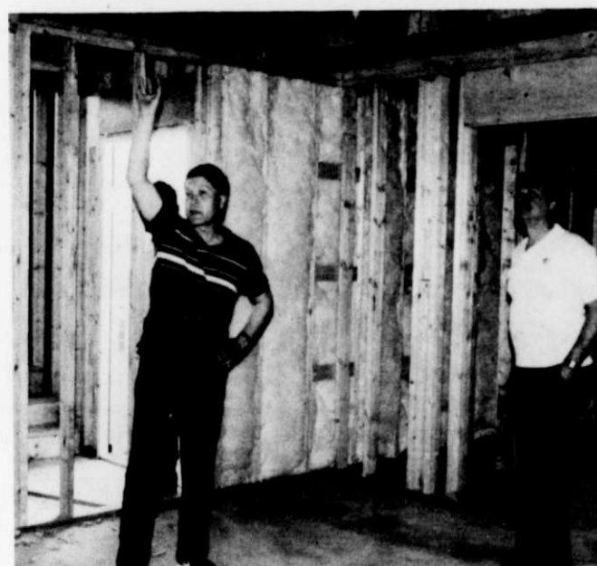
Bob Kirst, general contractor for Mapledale, explains some of the features being incorporated into the building.
