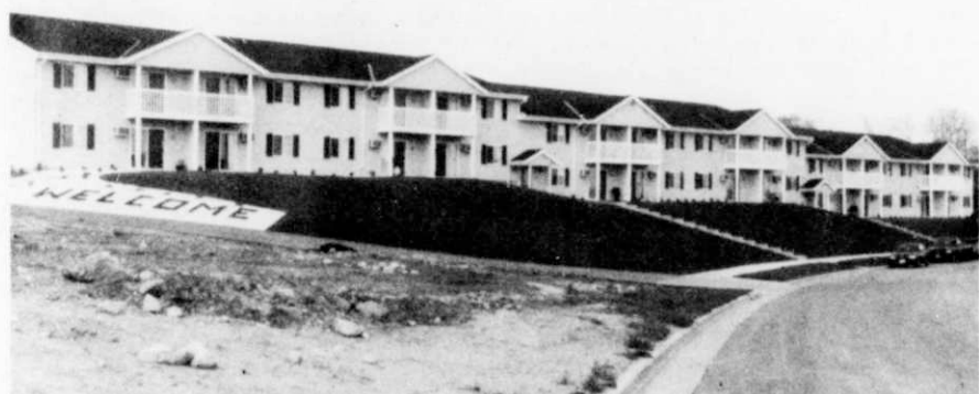
The 24-unit Rustic Timbers Townhouses, north of Kewaskum shopping mall, were recently completed and are 99% occupied.
