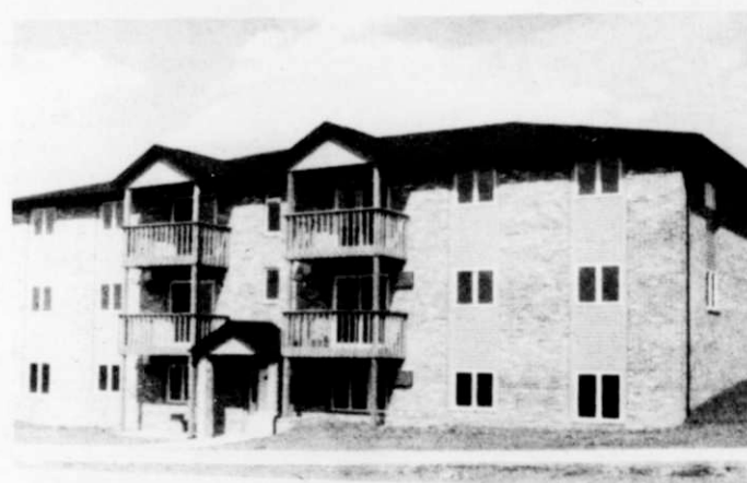
Westfield Apartments are located on the villages north side. Landscaping is all that remains to be done at the ten-unit building.
