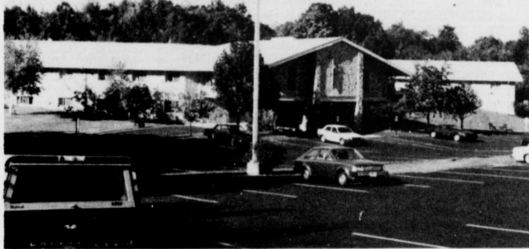
Cedar Lake Home's Friendship House, nestled among the campus' wooded hills provides skilled care for Alzheimer victims and those with related disorders.
