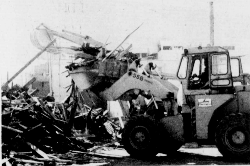
Loading up the debris.
