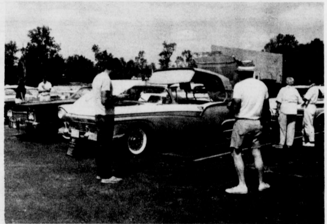
A rarity among cars is this 1957 Ford retractable hardtop convertible. The metal roof actually folds up and retracts to store in the car's trunk.
