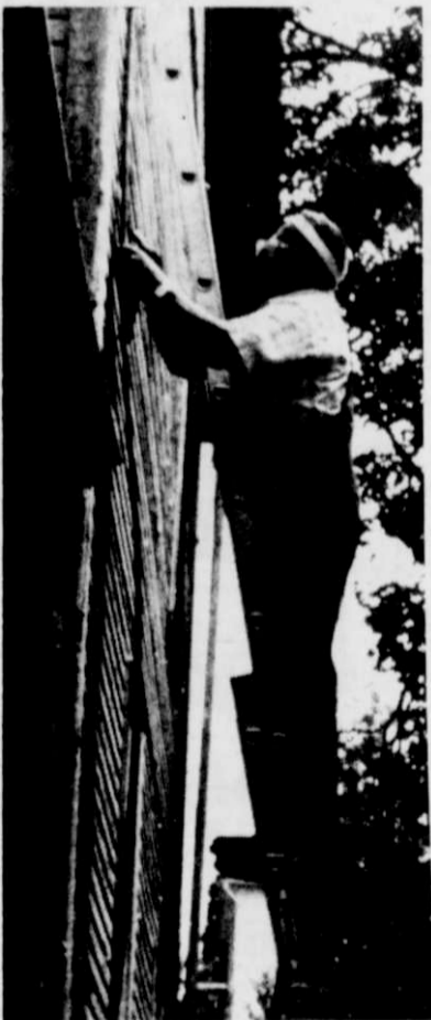
Willard Gruhle works on electrical wiring on Gallagher Street.
