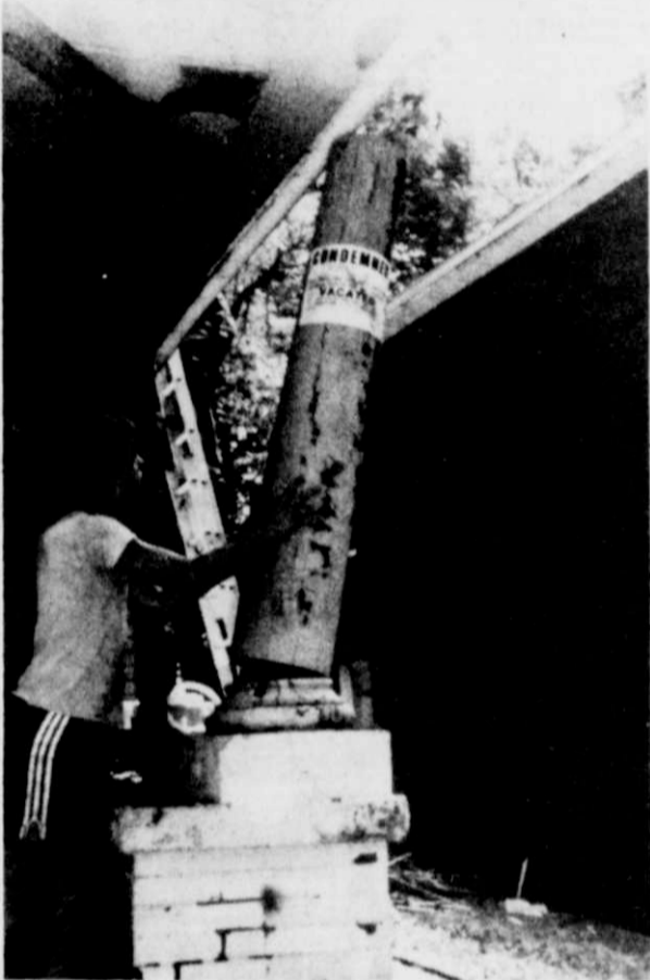
Robert Schreffler dismantles an old porch.
