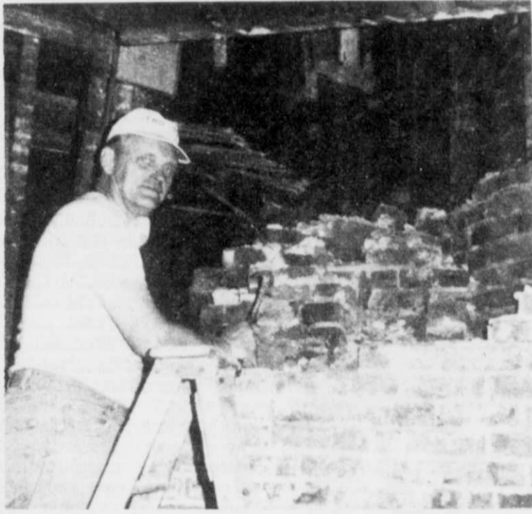
Rev. Bettin dismantles an old fireplace on Gallagher Street.
