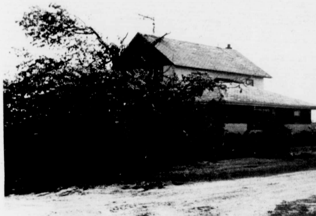
A large tree on the Jerry Herman farm, Hwy. W, narrowly missed the house when it was felled in last Wednesday night's storm but it did land on top of a car parked next to the home.
