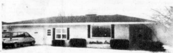
If you are looking for quality plus a beautiful location overlooking the river, then this is the home for you. Spacious all brick ranch, 2 natural fireplaces, main floor family room with patio plus built-in barbecue pit. Huge rooms, rec room lower level, 90 x 130 lot. K88
